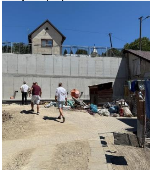
Obr. 4 Oporný múr v obci Dolné Semerovce. Fig. 4 Retaining wall in the village of Dolné Semerovce.
